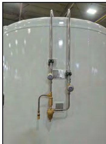
Photo 8 - Economizer Plumbing Circuit
