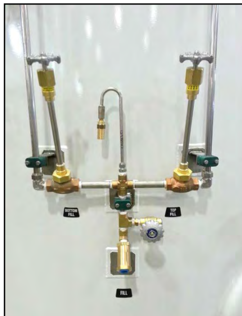
Photo 6 - Fill Circuit
